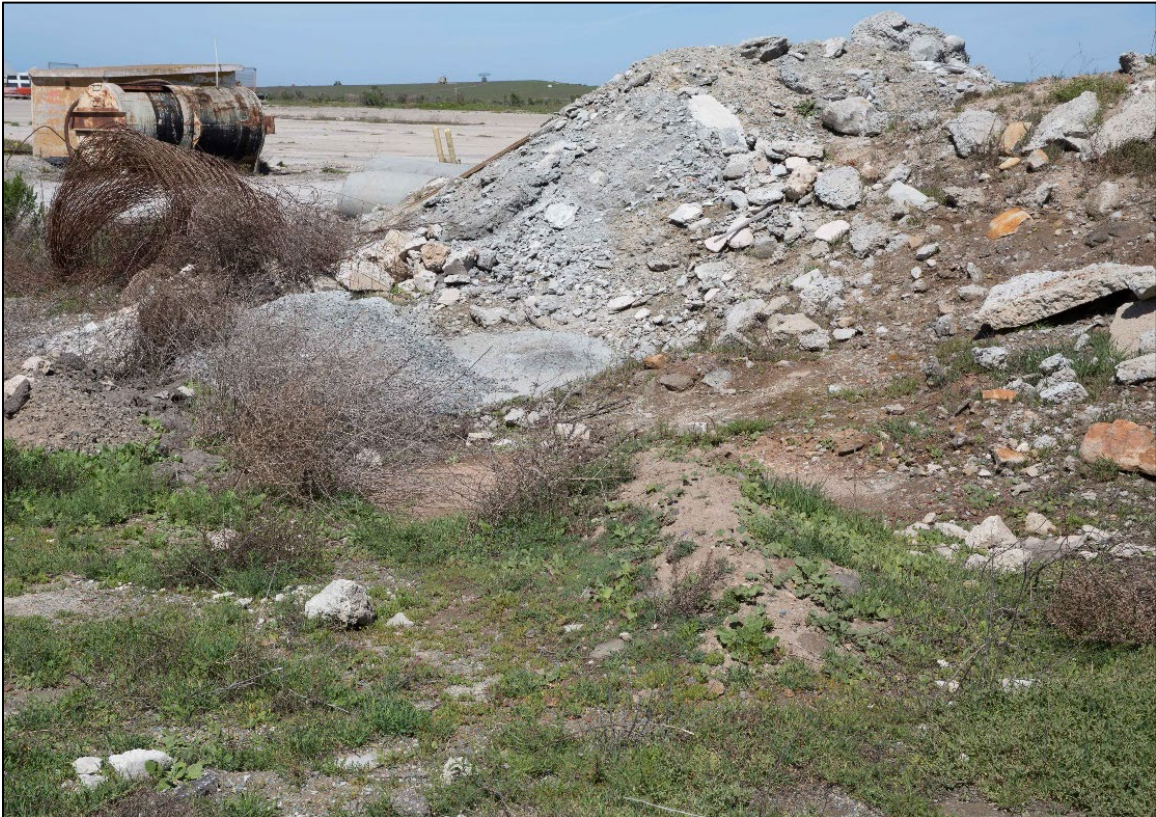
Figure 4-4. Example of stockpiling creep. Piles should maintain a 12-foot distance from all vegetation.
