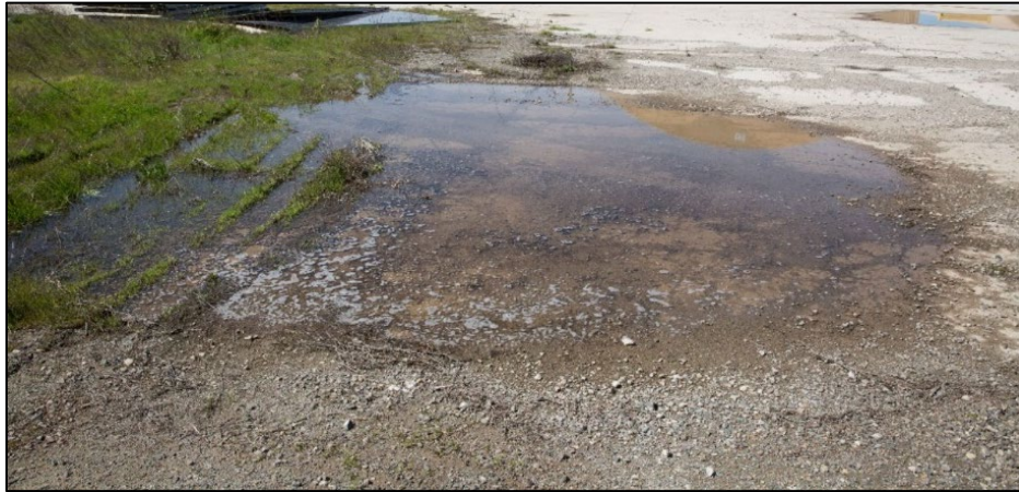
Figure 4-13. Pools of waters around infrastructure should be discouraged and surfaces should be regraded. This pool could encourage waterfowl to frequent the pond and subsequently introduce San Diego fairy shrimp ( Branchinecta sandiegoensis ) or other federally listed branchiopods (Muñoz 2013).
