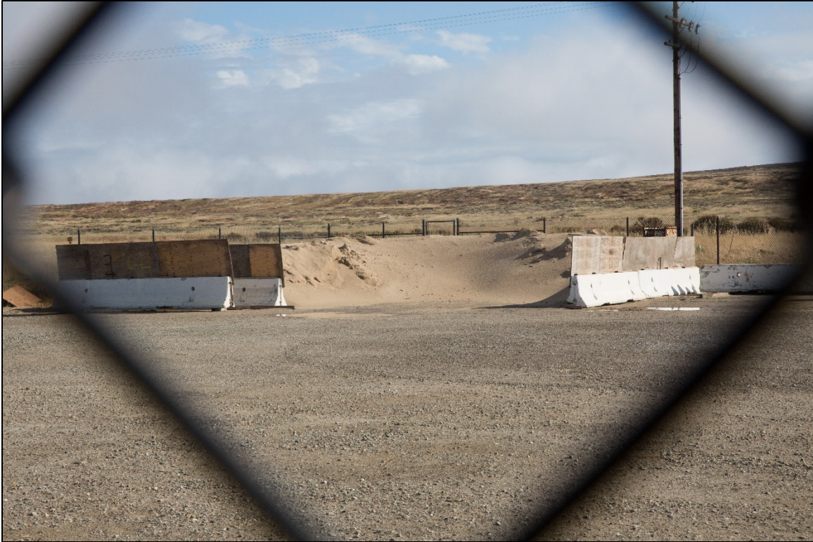
Figure 4-1. Stockpiles of sand, aggregates, or other materials should be treated with pre-emergent herbicides to prevent the transport of invasive plant species.
