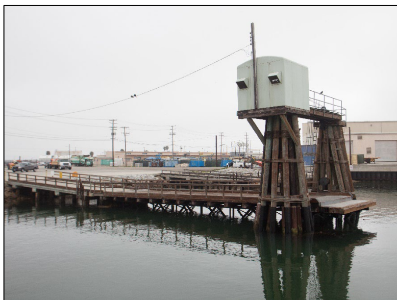
Figure 3-15. NBVC Port Hueneme barge loading area.
