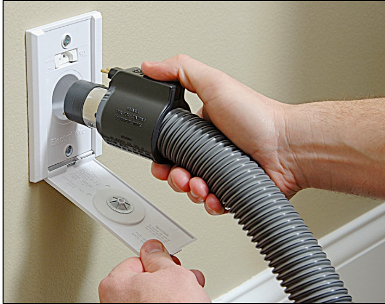
Figure 3-29. Example of a wall vacuum with a hose attachment that can be used to maintain cleanliness at the biosecurity station as well as to vacuum footwear and personal effects.
