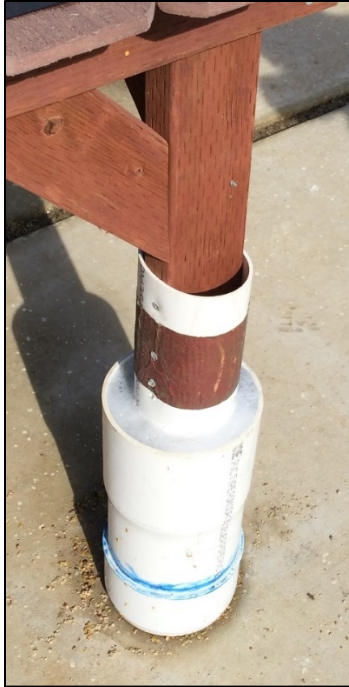
Figure 4-14. San Nicolas Island nursery table legs are adapted to prevent the infestation of Argentine ants in native plants starts, mosquito larvae, and the transfer of decollate snails. Designed by Channel Islands Restoration.
