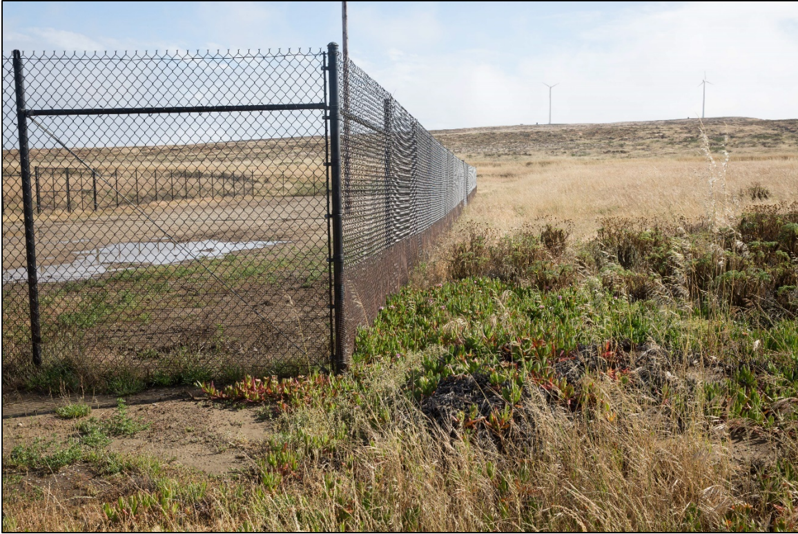
Figure 4-3. Example of a yard that would benefit from a 12-ft (3.7 m) gravel buffer and pre-emergent herbicide treatment.
