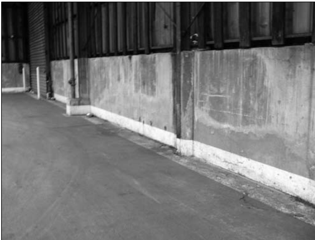
Figure 3-23. Rats leave rubbings (dark greasy stains) along linear locations, usually between a nest and food source. Painted white rat runs will enable management to determine if integrated pest management trapping efforts are successful.
